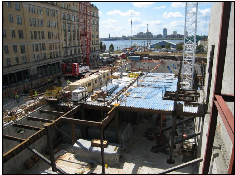
Figure 8: Locations of the crawler & tower cranes. Photo taken by Vincent A. Rossi.
