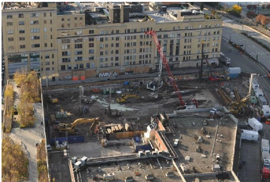
Figure 7: View of the MMAA excavation from the North. Note the puddles throughout the site. Photo courtesy of the Metro Museum of American Art.
