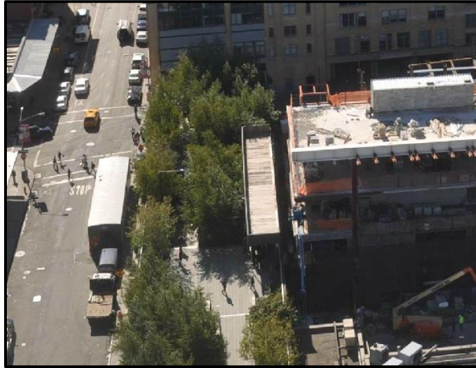
Figure 9: View of the overhead protection above the highline. Image courtesy of the Metro Museum of American Art.
